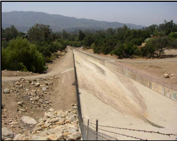
Photograph 53 (left). Stewart Canyon Creek showing aboveground flood control concrete channel (27 May 2004). Photograph 54 (right). Fox Canyon Barranca showing meander pattern in concrete channel (9 January 2005).
