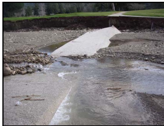
Photograph 51 (left). San Antonio Creek Arizona Crossing at Soule Park Golf Course creating a major barrier to Steelhead (16 July 2004). Photograph 52 (right). San Antonio Creek Arizona Crossing at Soule Park Golf Course was washed out and buried by sediment during significant winter storm (8 February 2005).
