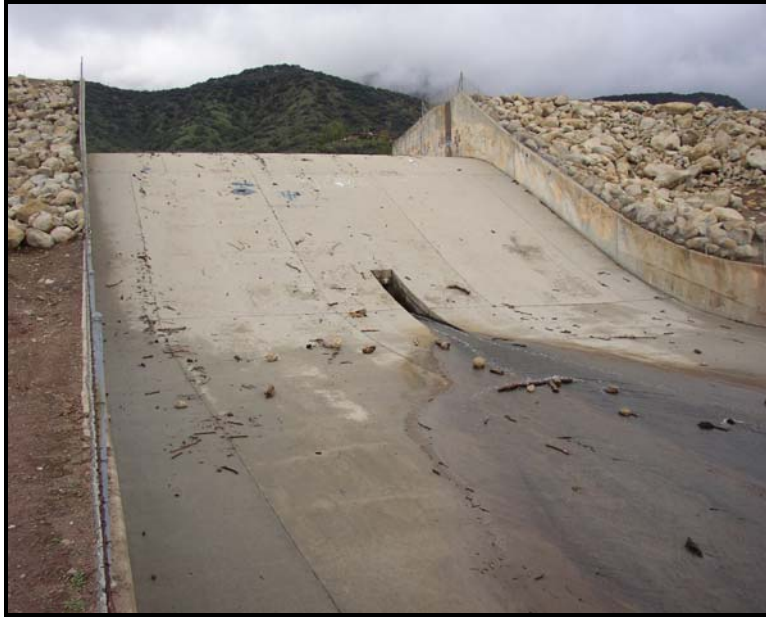
Photograph 88. Stewart Canyon Debris Dam Spillway (28 January 2005).
