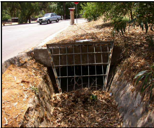
Photograph 55 (left). Undergrounding of Ojai Creek (27 May 2004). Photograph 56 (right). Undergrounding of Stewart Canyon Creek by a flood control channel and box culvert (8 January 2005).
